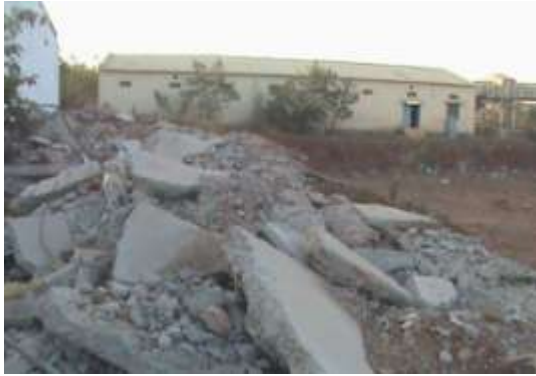
Fig.1 Collection of demolished concrete waste
