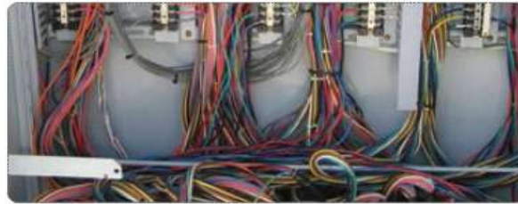
Fig 6. Many Connections Need To Be Made In Each Apparatus In The High Voltage Equipment Switchyard
