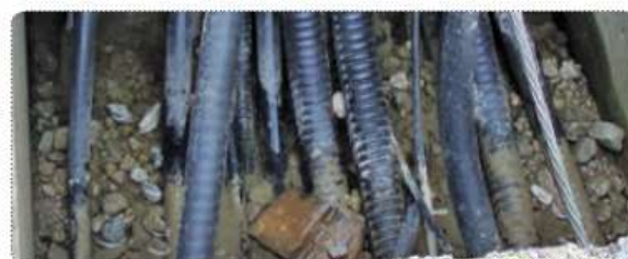
Fig 5. Extensive Amounts Of Copper Cables Need To Be Distributed From Each Switchyard Apparatus Back To The Control House
