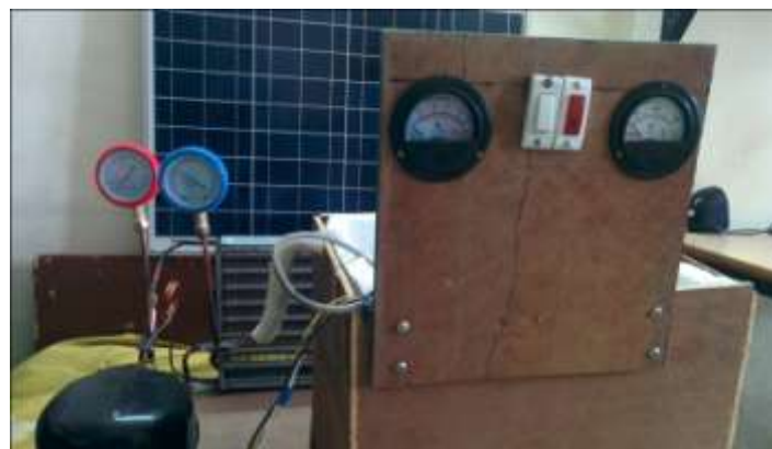
Figure 2: VCRES system assisted with solar power
