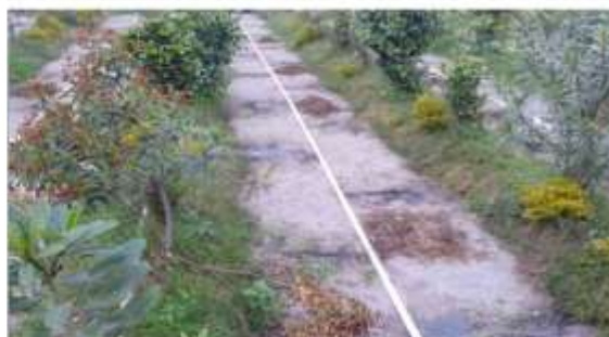
SBT Plant at Lucknow Airport
