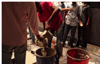
Fig. Shows the Mixed foam concrete for Density measurement.
