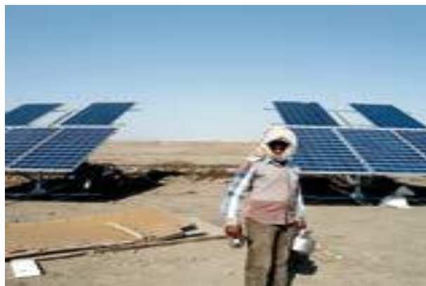
Pic.2: Solar Pump Installed in Gujrat ^
