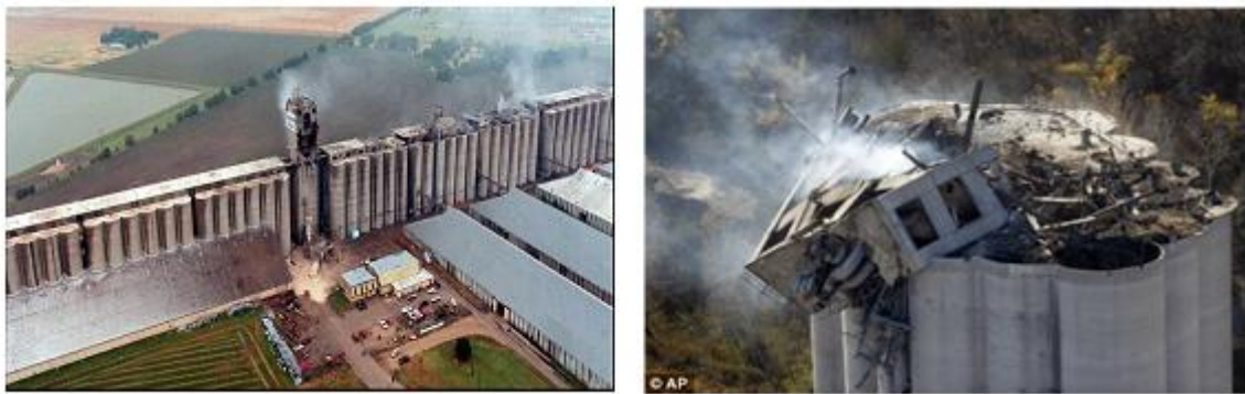
Fig.1.3 View of the damage to DeBruce Grain Elevator
