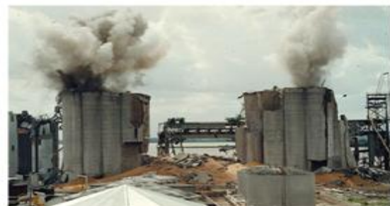
Fig.1.2 View of the damage caused by the Blaye explosion
