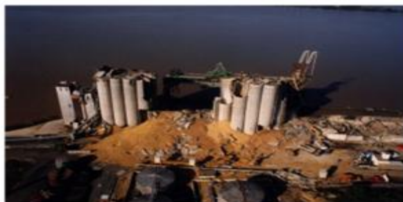
Fig.1.2 View of the damage caused by the Blaye explosion
