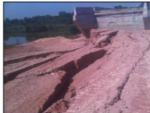
Site Photo of Embankment failure (Sliding & Shear) for Additional Embankment toe width
