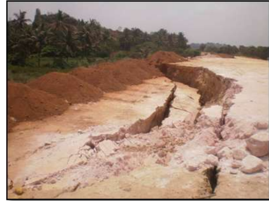
Site Photo of Embankment failure for Additional Embankment toe width
