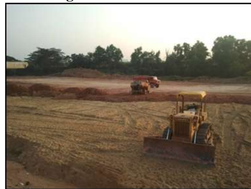
ix) Construction of embankment with compacting in layers of 200mm thick using good quality lateritic soil.
