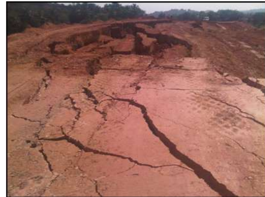
Site Photo of Embankment failure for Additional Embankment toe width
