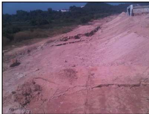
Site Photo of Embankment failure (Sliding & Shear) for Additional Embankment toe width
