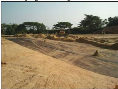
ix) Construction of embankment with compacting in layers of 200mm thick using good quality lateritic soil.
