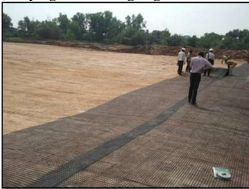
viii) Laying of drainage blanket of 0.45m thick consisting of clean sand.
