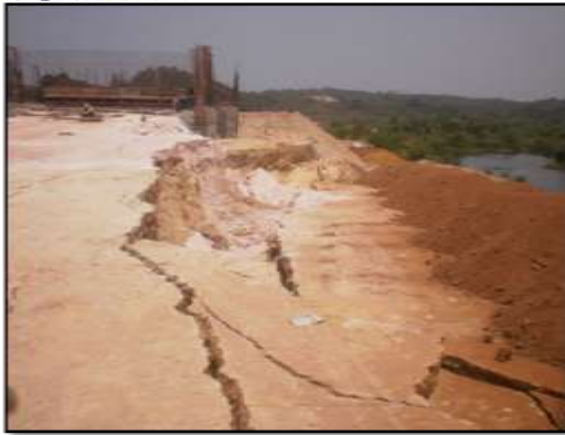
Snapshot after embankment failure after additional widening of the base
