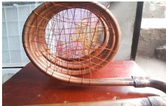
Fig.8 installing coiled tube in tank
