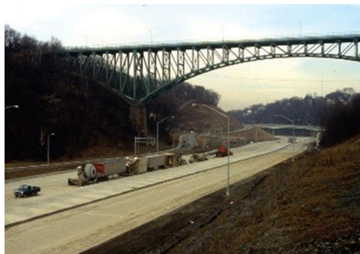
Figure 4: Fly Ash Utilization in Fills/Embankments (Courtesy: ACAA)
