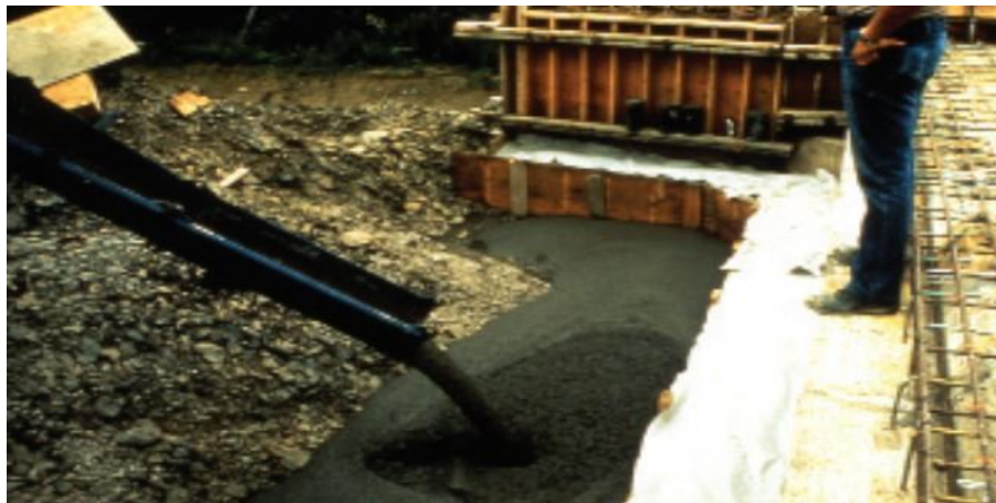
Figure 3: Bridge abutment backfill with flowable fill (Courtesy: ACAA [28]).
