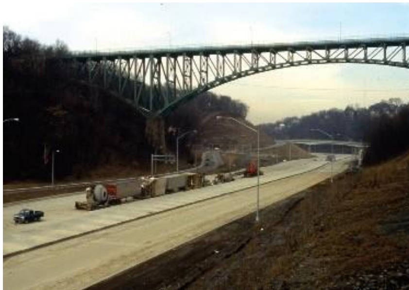
Figure 4: Fly Ash Utilization in Fills/Embankments (Courtesy: ACAA [28])
