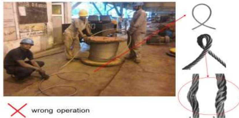
Fig.1: Unsafe Situation Without Using Wire Rope Uncoiling Stand
