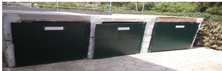
Figure 3. View of model buildings constructed for thermal study
