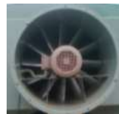
Figure 1.8: Single -Stage Axial Flow Fan
