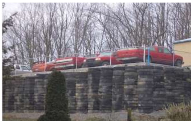
Fig.8. Confined Aggregate Concrete as a Retaining wall
