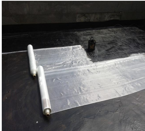
Fig 5: Fiber Mesh with Overlapping
