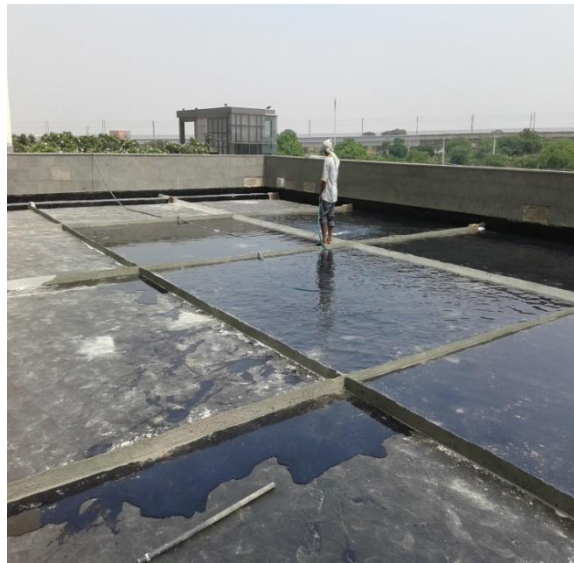
Fig 6: Testing of Seepage after Treatment
