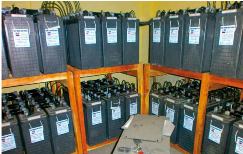
Fig.2.Battery Bank Installed to Store Solar Power
