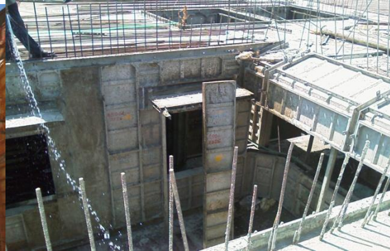
Wall formwork in position with window openings
