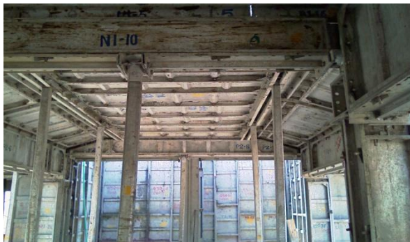
Slab & beam support formwork
