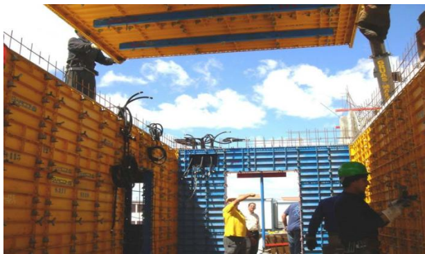
Wall formwork in position with door openings
