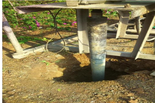
Fig. 2.3.1 Drilling Of Bore Hole
