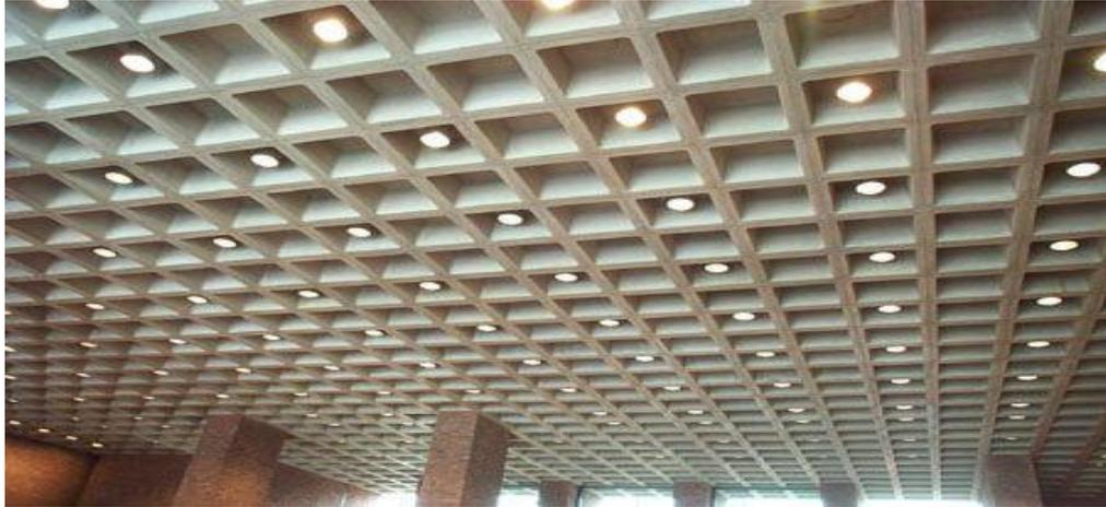
Figure 3: Grid Slab [10]
